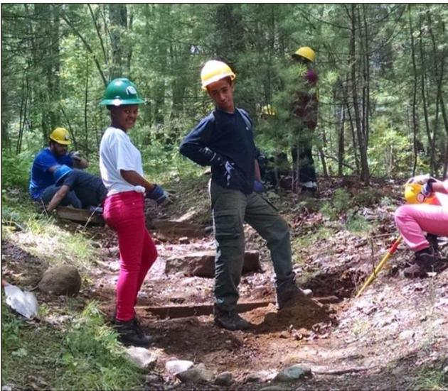
➤ *Old Colony YMCA crew hard at work on check steps and waterbars to address erosion on a popular BCT spur trail.*
